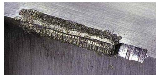
Repair corner areas
